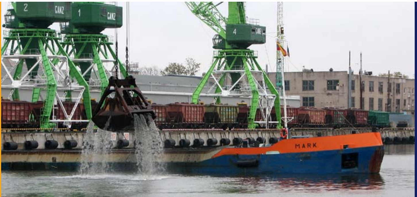
Dredging of sediments in Klaipeda port (photo by E.Visakavičius)
